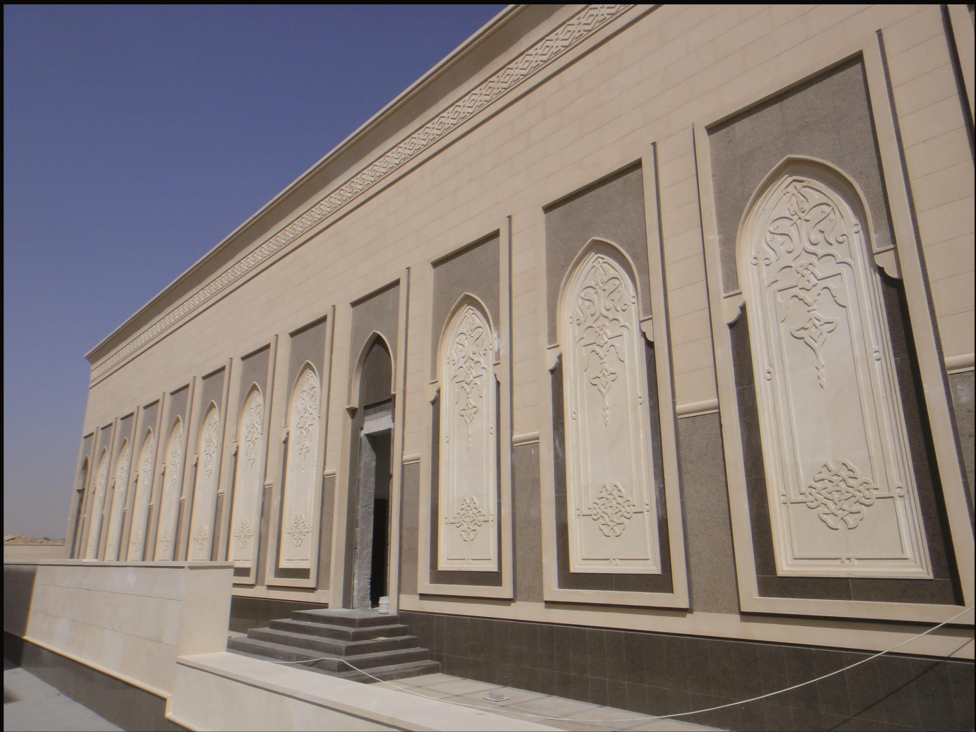
The external facades are decorated with GRC panels decorated with botanical motifs inspired by the windows, and the external formation of the facades is closed with a cornice that contains geometric motifs.
